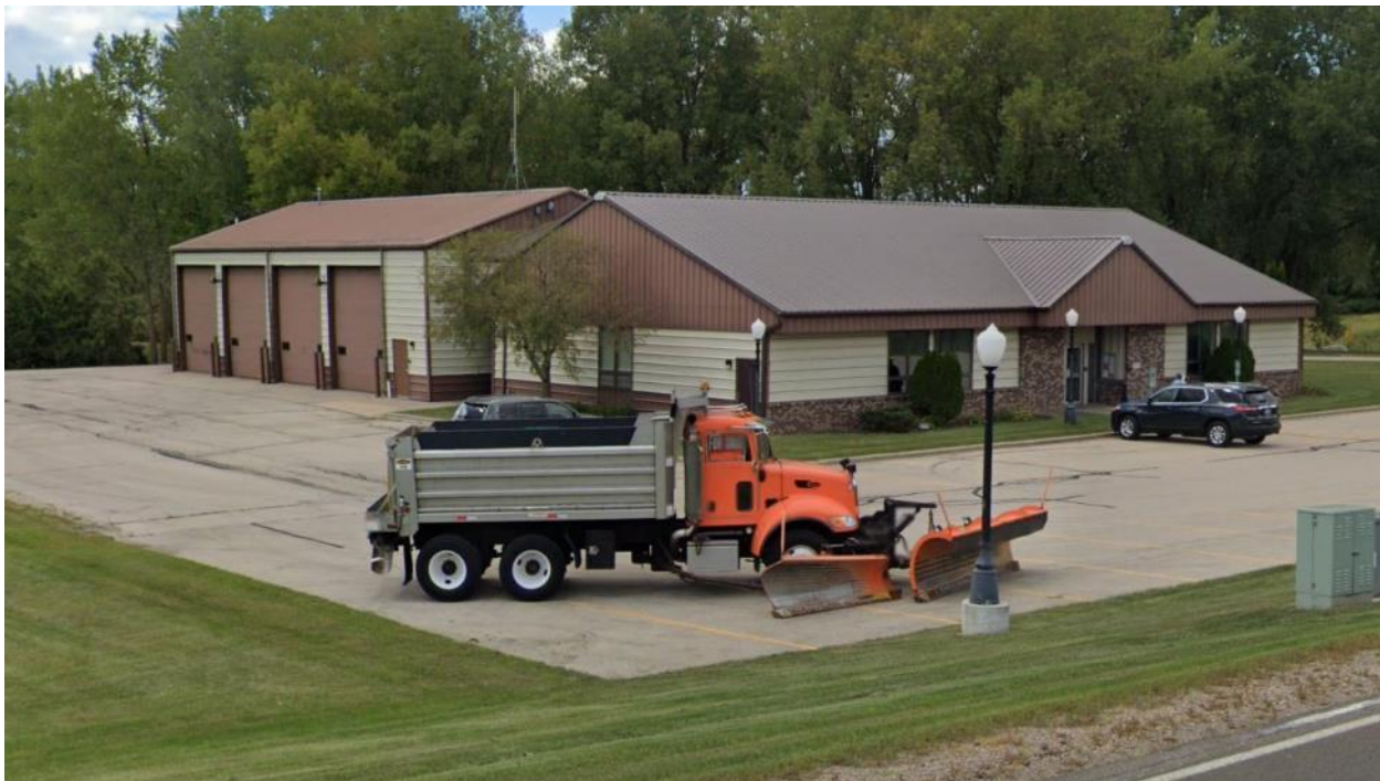
Town of Burke Town Hall and Garage.
