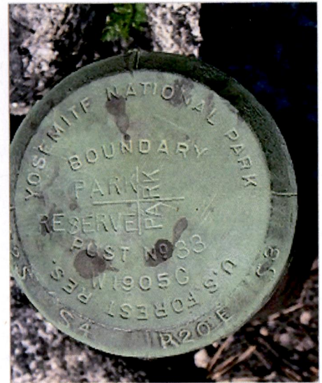
Figure 4. The cast and stamped cap on a corner monument pipe, in western Yosemite National Park, placed in 1905 during the Park boundary resurvey.
